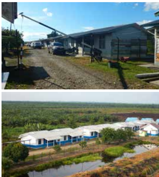
/// Renovation of the staff housing at the Dendymarker Indah Lestari (DIL) mill, photos before and after ///
