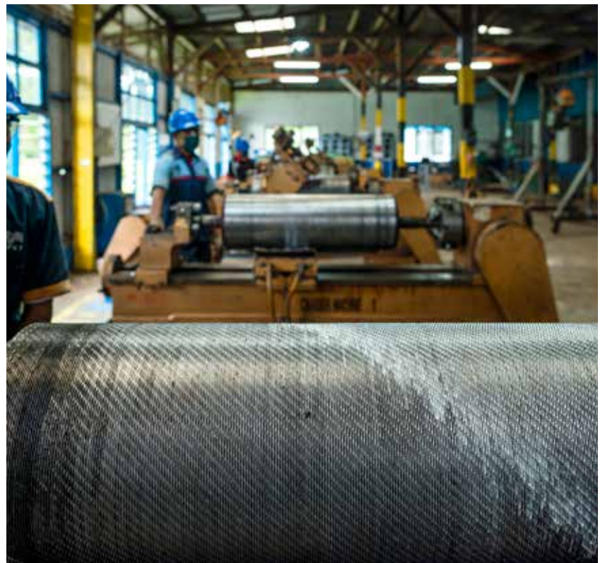
/// Workshop for the maintenance of the cylinders of the CTC machines (‘Cut, Tear and Curl’) ///
