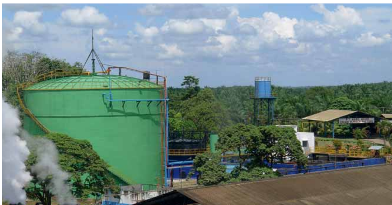
New generation methane capture system at Mukomuko POM, Indonesia.
