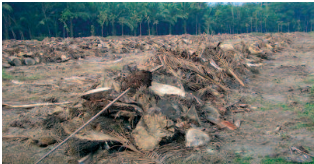
Felled and shredded trees
