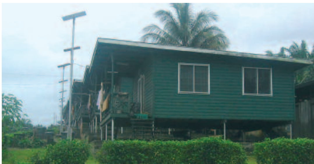
Solar panels at Kerakera - Hargy
