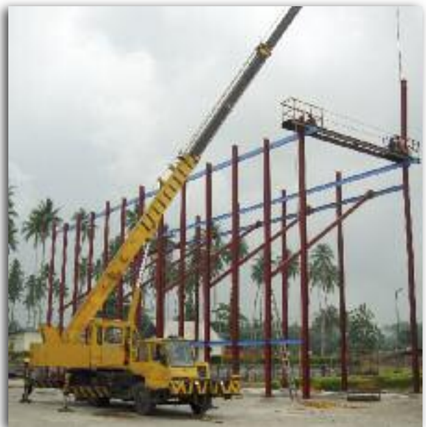
Construction works at Hargy - PNG
