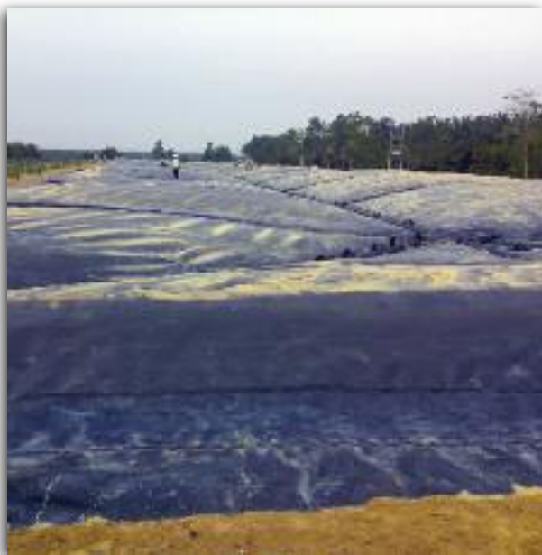
Methane gas capture
