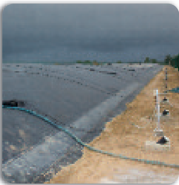
Covered lagoon for methane capture (Perlabian- Indonesia)
