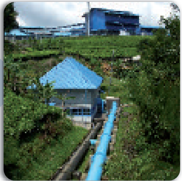
Hydro power station (Cibuni-Indonesia)
