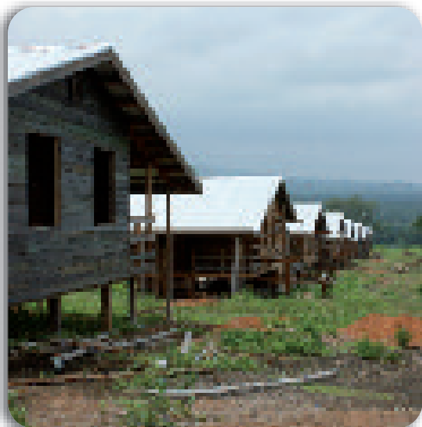
Labour houses under construction (Navo-PNG)
